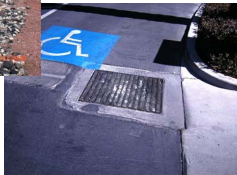
Sediment Deposit at Points of Flow Interception
