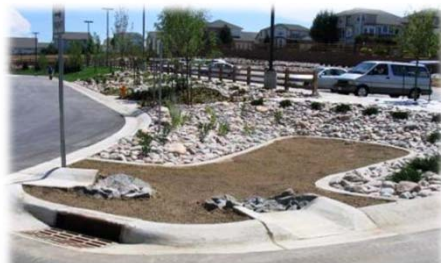
Construction of LID Rain Garden
