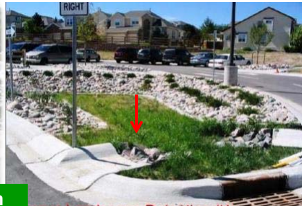
Construction of LID Rain Garden
