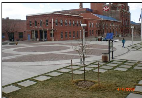
Porous Pavements in UC-Denver Campus
