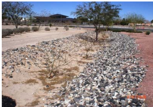
Sediment Deposit at Points of Flow Interception
