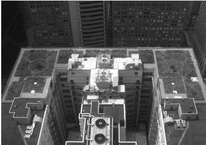
FIGURE 2.5 Green roofs, like this one on City Hall in Chicago, are good examples of multiobjective building techniques, by serving both natural hazard mitigation as well as climate change mitigation purposes. The vegetation captures excess rainwater while also cooling the building, thereby reducing the building's energy consumption.
